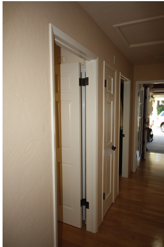
FIGURE 2.18 Expanding hinges and lever handles in Valinda Martin’s home.
