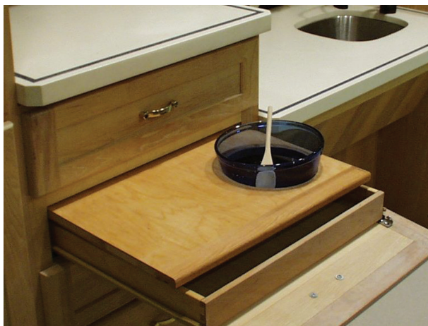
FIGURE 3.29 Within a raised cabinet in the GE Kitchen in the Center for Real Life Kitchen Design at Virginia Tech, the pull-out board has a cutout that holds a bowl steady for a person with limited dexterity or arm strength.
