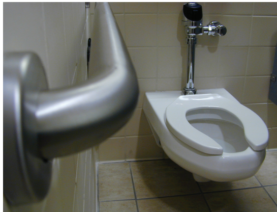
FIGURE 3.44 Each stall has grab bars of various heights, USC bathroom remodel.
