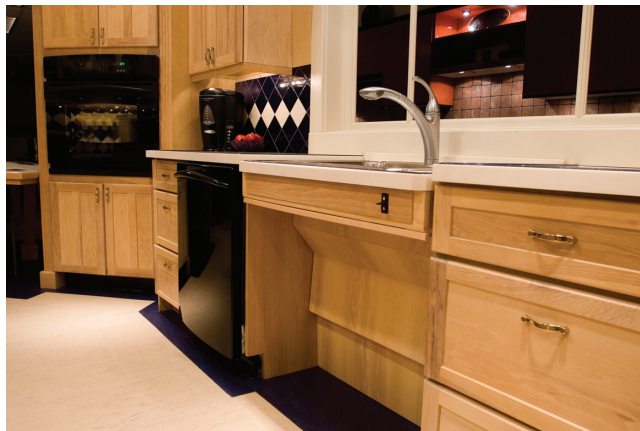
FIGURE 3.27 An adjustable-height sink with knee space, a single wall oven at counter height, contrasting counter edging and flooring.
