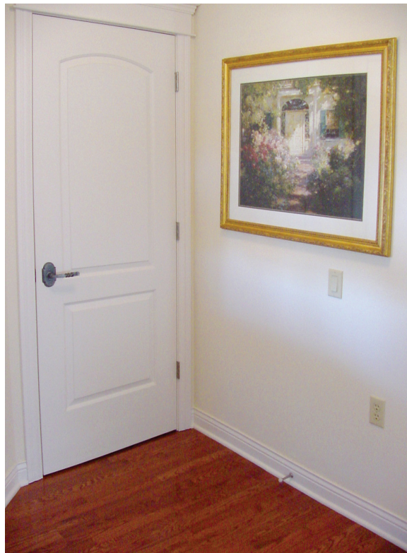
FIGURE 8.26 Kennedy house, entrance interior, lever door handle, and flat threshold.
