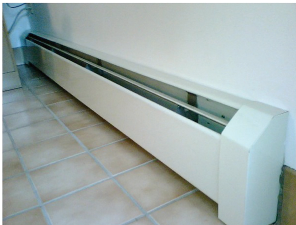
FIGURE 10.3 Radiant heated baseboard units eliminated the need for forced air vents in Ecology House (the generator is in another building).
