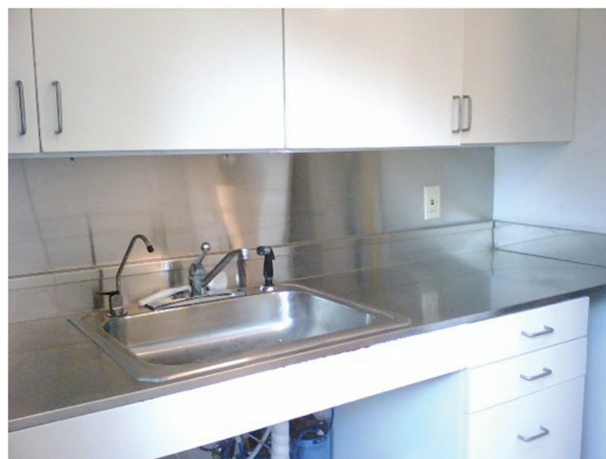
FIGURE 10.5 In kitchens, metal cabinets feature a baked-on surface and stainless countertops, sinks, and so on.
