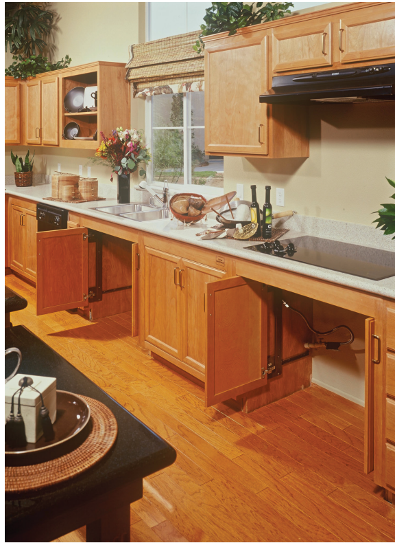
FIGURE 8.22 Accessible cabinets by Susan Mack, OT; cabinet doors are retractable. Note the finished floors under both sink and range cabinets.
